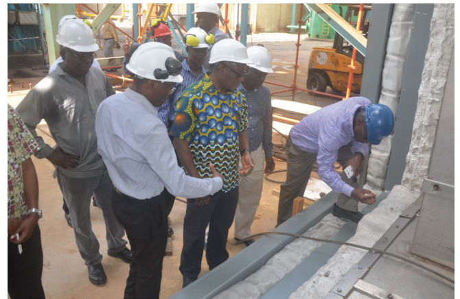
Ing. Badger inspecting the project
